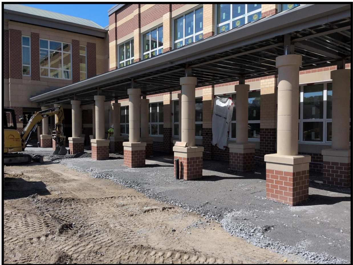
Final grading at main entrance canopy – 06/04/26
