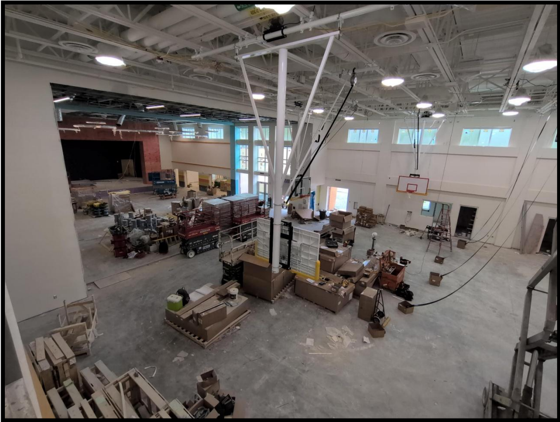
Gym equipment installation progressing – 05/07/26
