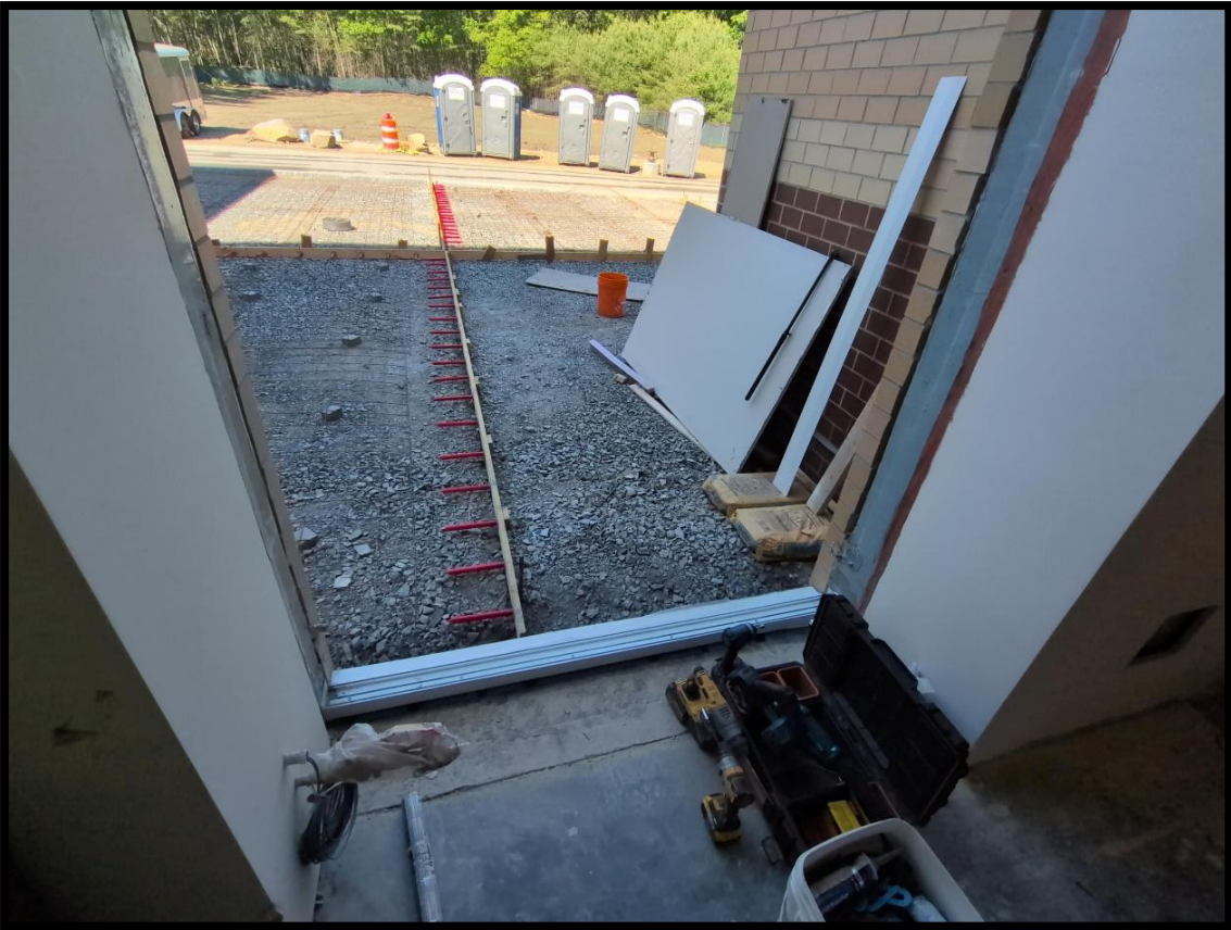
Storefront frame installation at cafeteria north wall – 6/04/2026
