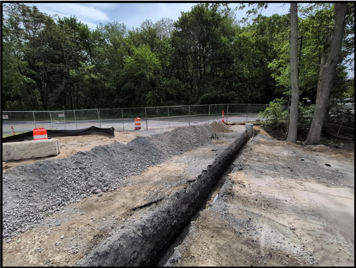
Conduit and light pole bases installed – 06/03/26
