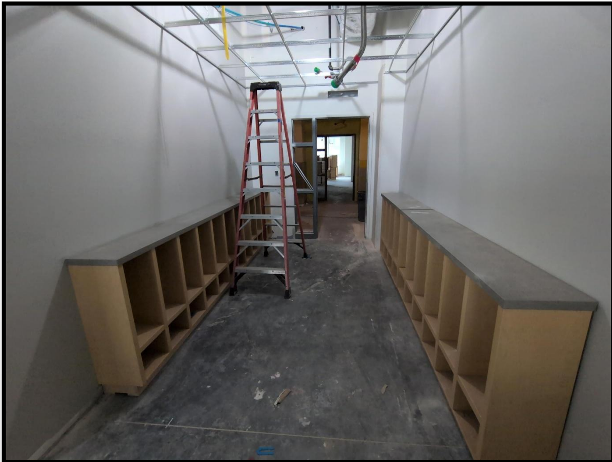
Cubbies installation progressing at B-1 – 05/06/26
