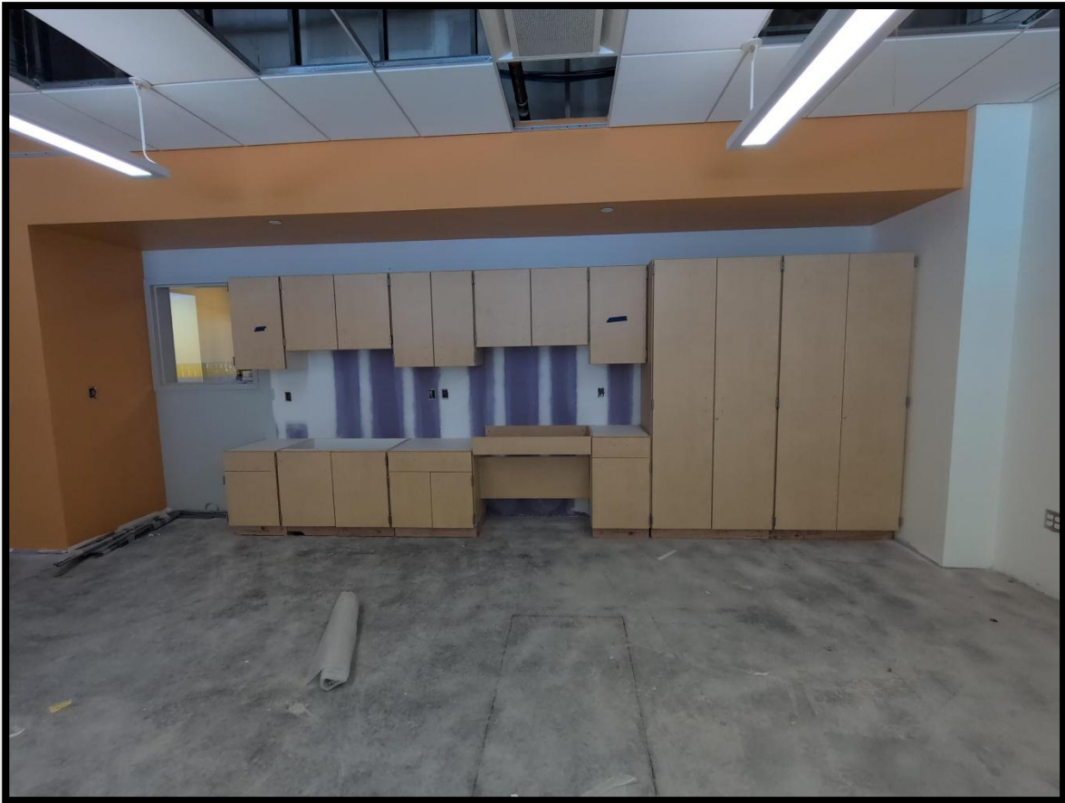
B-2 cabinets installation progressing – 06/03/26
