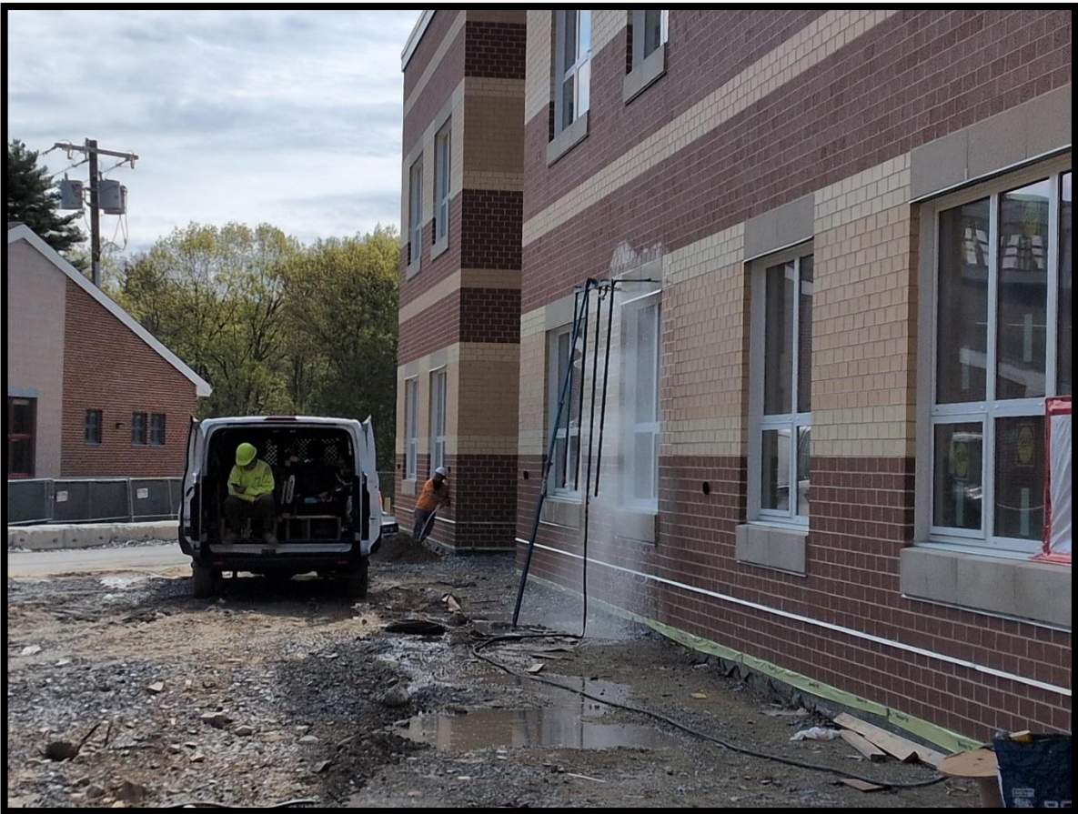
Window testing at C-1 east wall – 05/11/26
