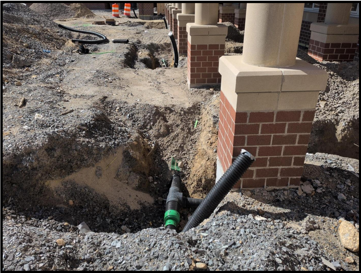
Drainage installation at main entrance canopy – 06/03/26
