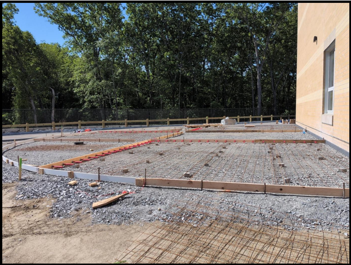
Exterior classroom concrete forms in place south of C wing – 06/03/26
